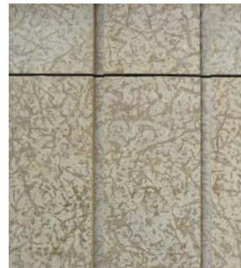
**Figure 5.** Tyndall stone showing fossil remains and characteristic mottling.
