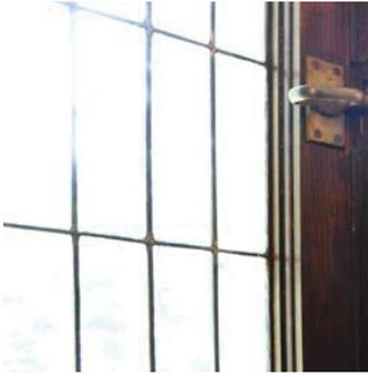
Figure 17. A leaded glass window; lites separated by lead glazing bars.
