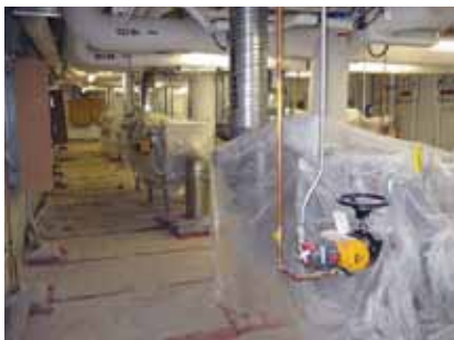
HEPA filters for CL-3 Labs
