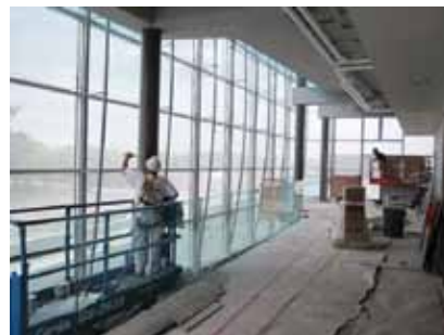
Working on the first floor mixing chamber
