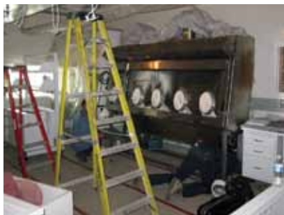
Installing the biosafety cabinets (gloveboxes)
